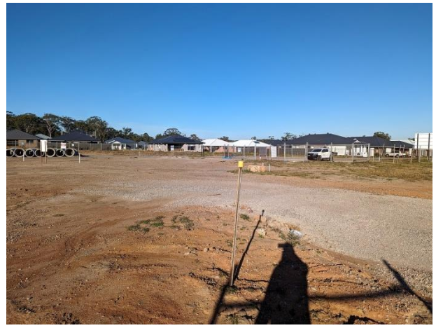
Photograph 6: From near eastern boundary of Lot 611, facing southwest.
