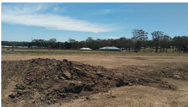
Photograph 3: From near eastern boundary of Lot 503, facing northwest.
