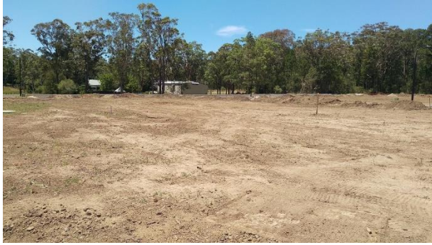
Photograph 5: From near south-western corner of Lot 507, facing north-northeast.
