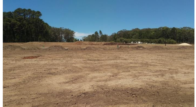
Photograph 6: From near south-western corner of Lot 507, facing east.
