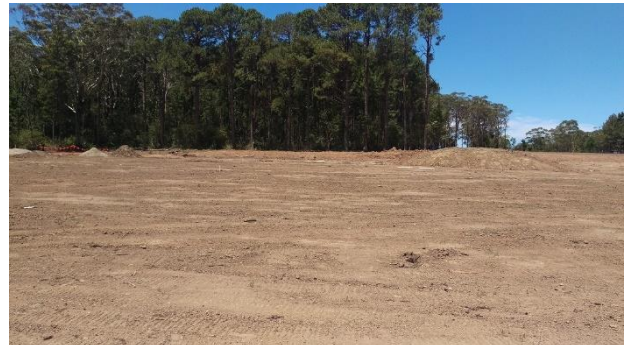
Photograph 8: From near south-western corner of Lot 510, facing east.
