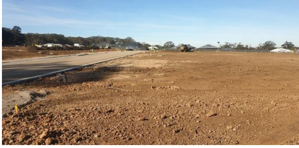
Photograph 5: From near north-eastern corner of Lot 410, facing south.
