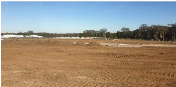
Photograph 9: From near eastern boundary of Lot 415, facing east.
