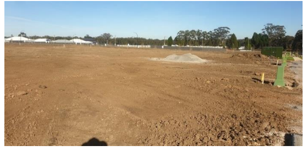
Photograph 6: From near north-eastern corner of Lot 410, facing west.
