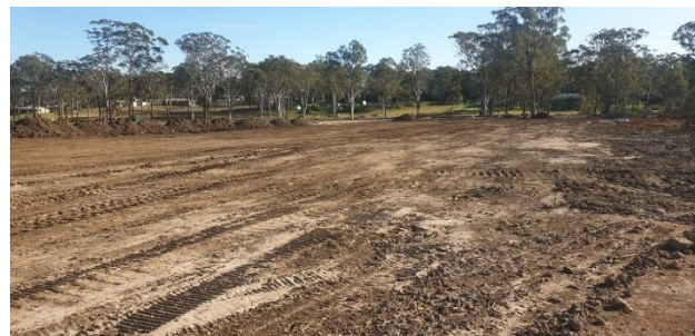
Photograph 12: From near eastern boundary of Lot 418, facing north.
