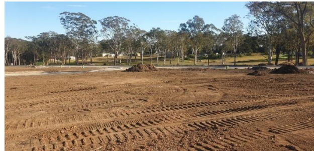
Photograph 10: From near eastern boundary of Lot 415, facing north.
